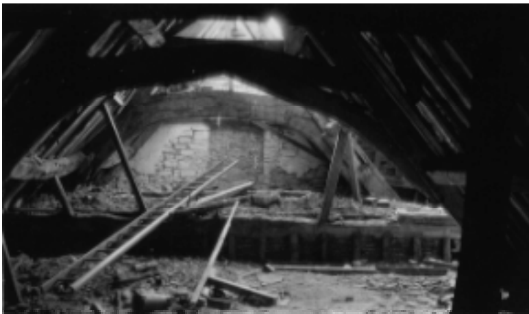
Repairs to medieval cruck roof in east wing by Norman Jewson in 1925-6
